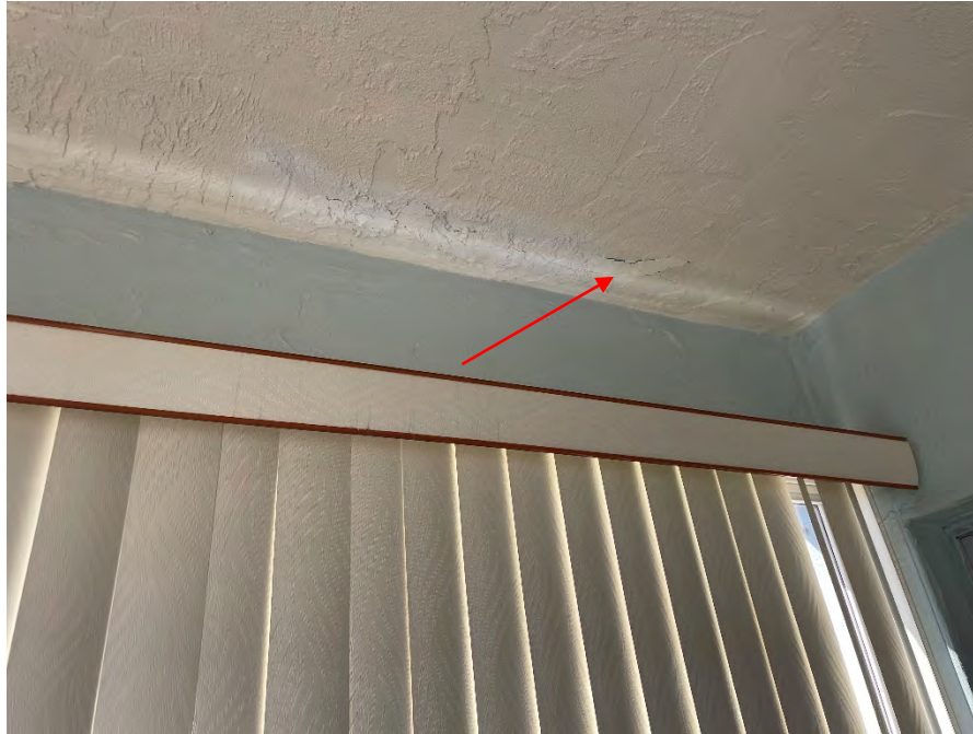
Figure 27 - Cracking in ceiling of unit J203
