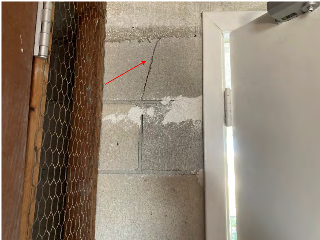
Figure 32 - Cracking in CMU wall in storage room
