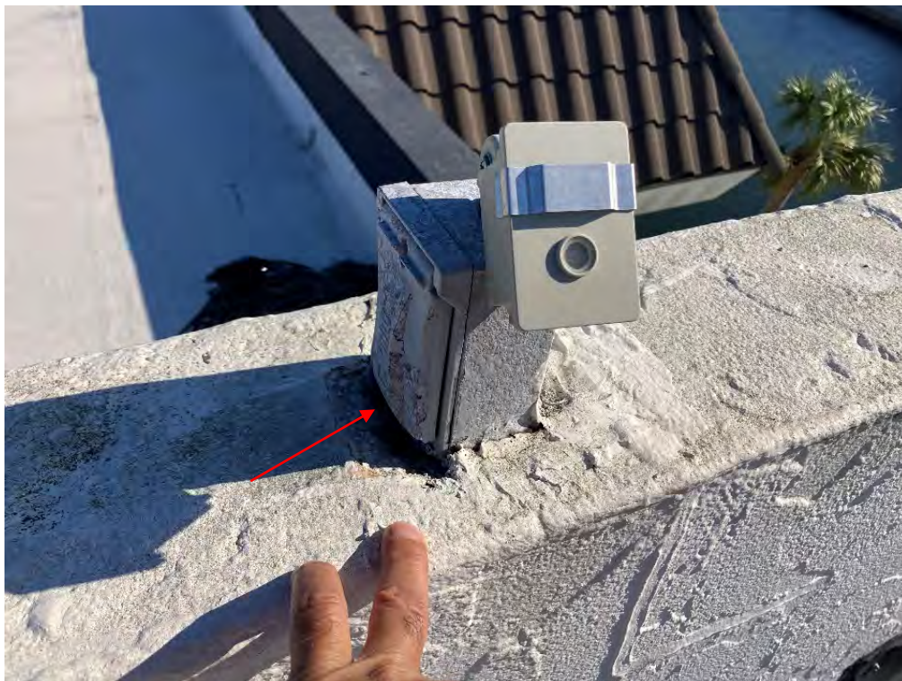
Figure 30 - Extrusion to be sealed properly
