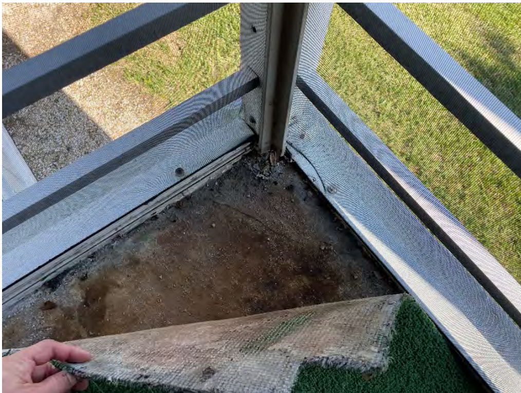
Figure 18 - Water damage under carpet of Unit F201
