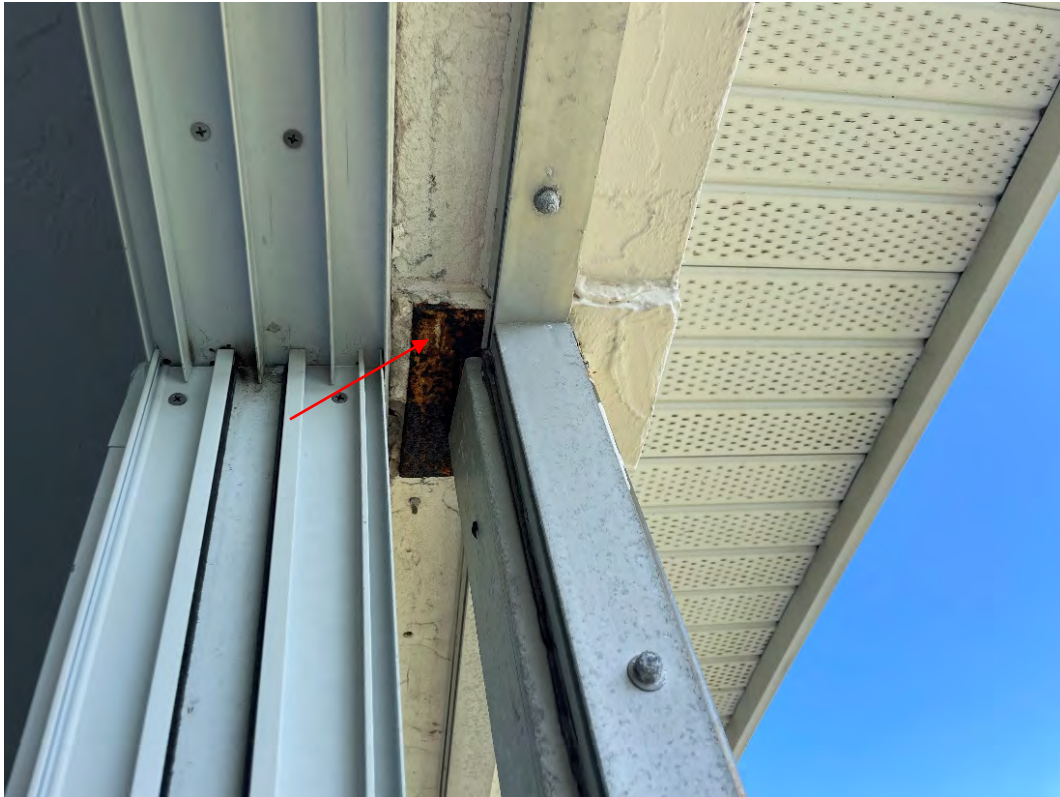
Figure 17 - Rusted connection plate by window of Unit F308
