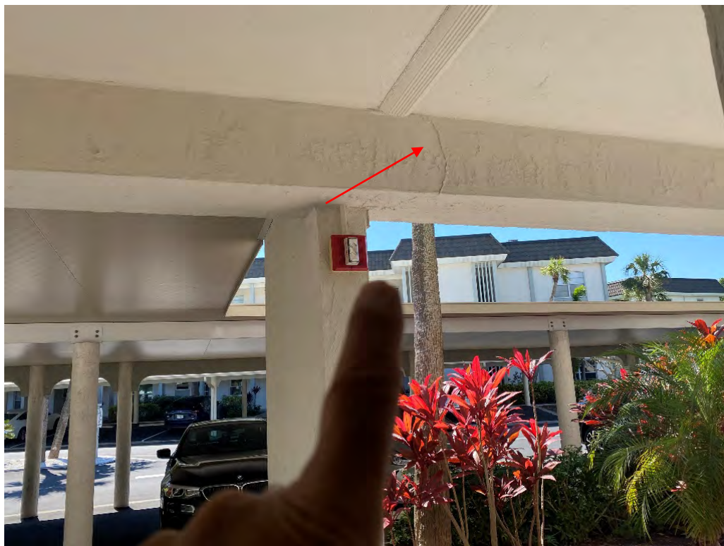
Figure 46 – Surface cracking on beam on the underside of level two
