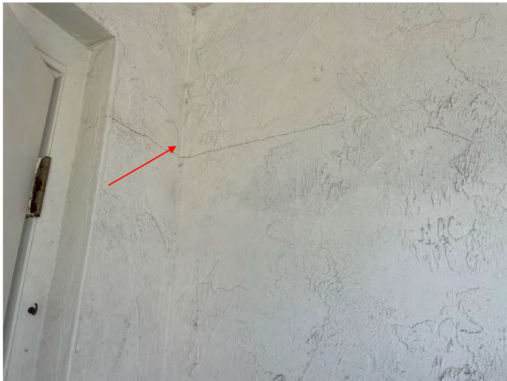
Figure 22 - Stair-stepping in Unit G306
