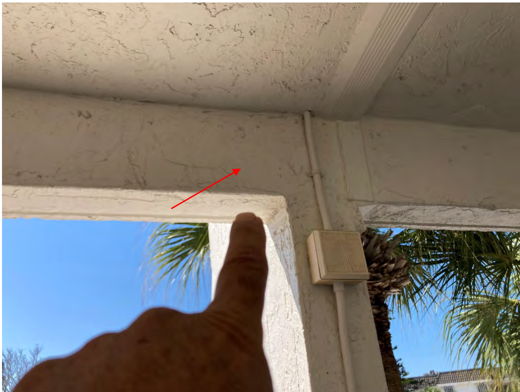
Figure 38 - Cracking on beam on level three
