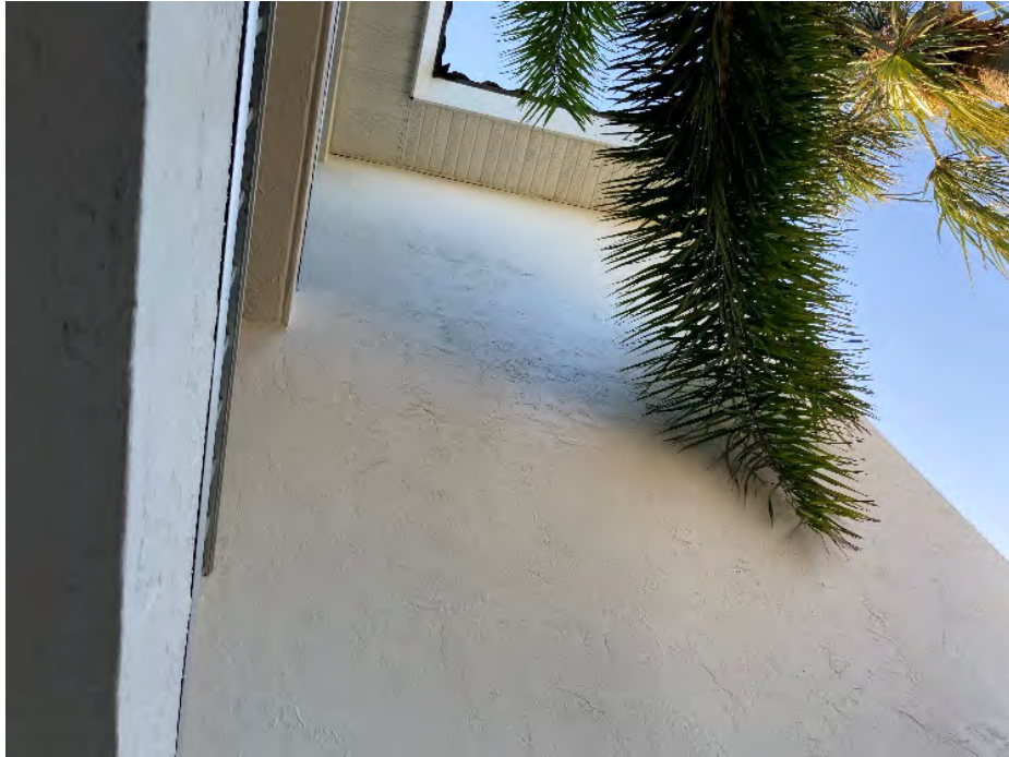
Figure 7 - Plants rubbing against exterior wall, typical
