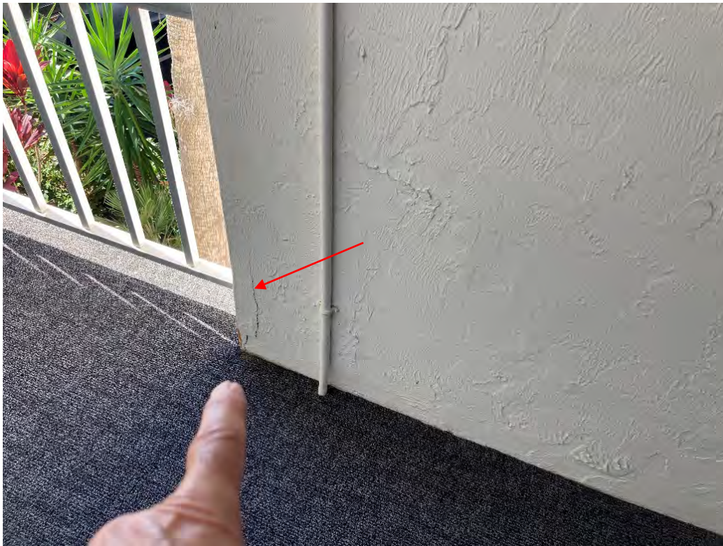
Figure 43 - Cracking in wall on level two
