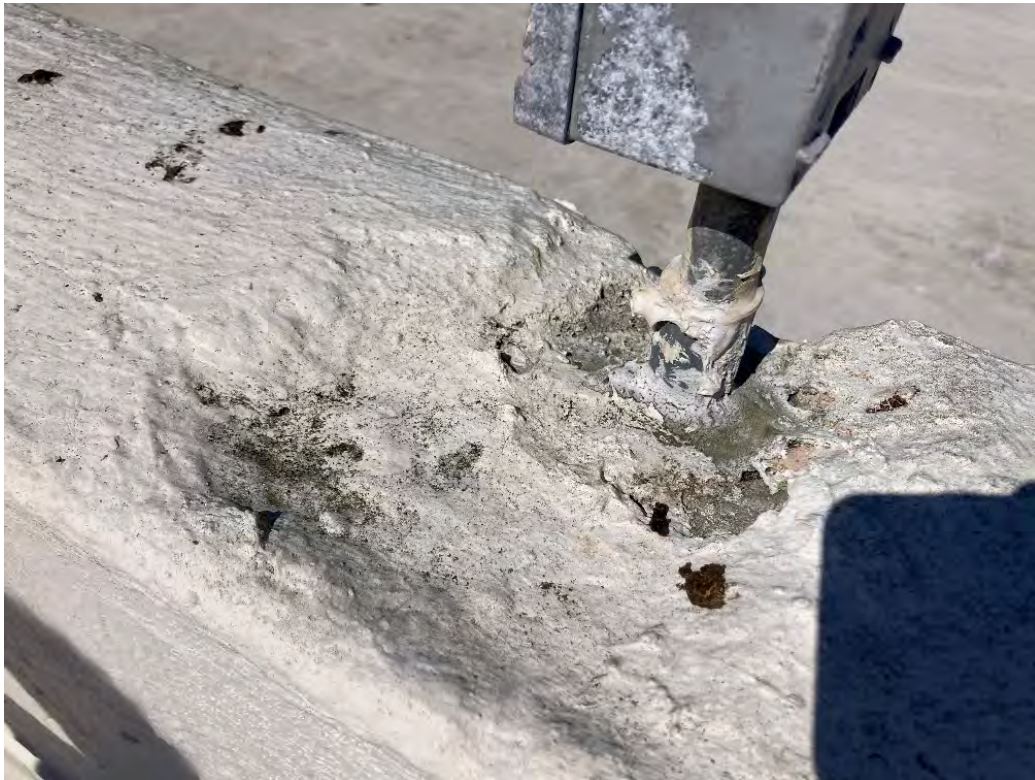
Figure 40 - Extrusion not properly sealed
