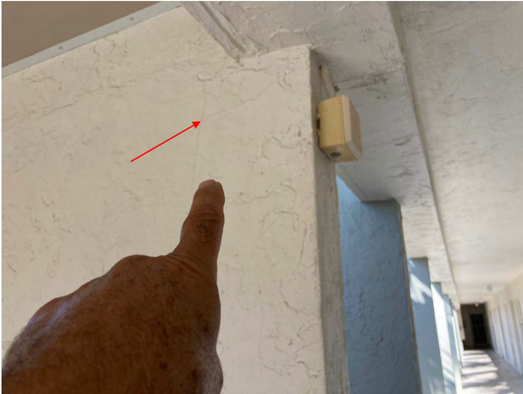
Figure 37 - Cracking on column on level one
