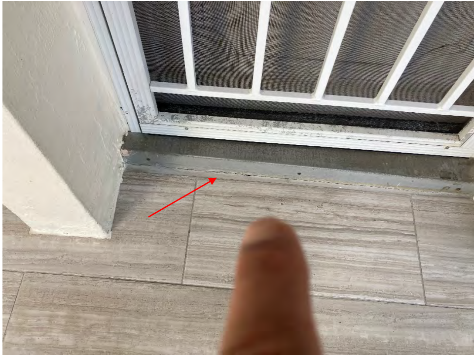
Figure 15 – Cracking sealant in front of Unit E105
