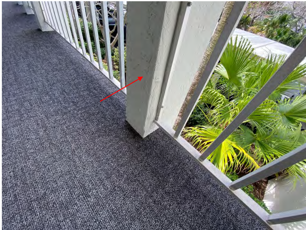
Figure 16 - Cracking in stucco on column on 2 nd floor walkway
