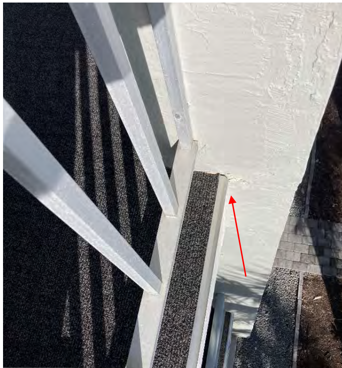
Figure 26 - Paint delamination on column on level three
