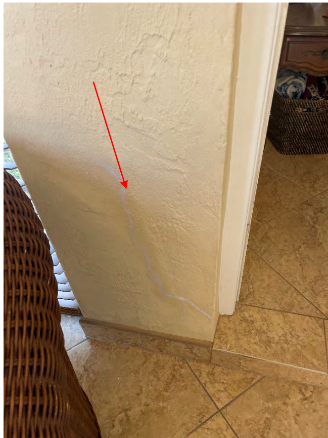
Figure 28 - Crack chased with sealant in Unit 108
