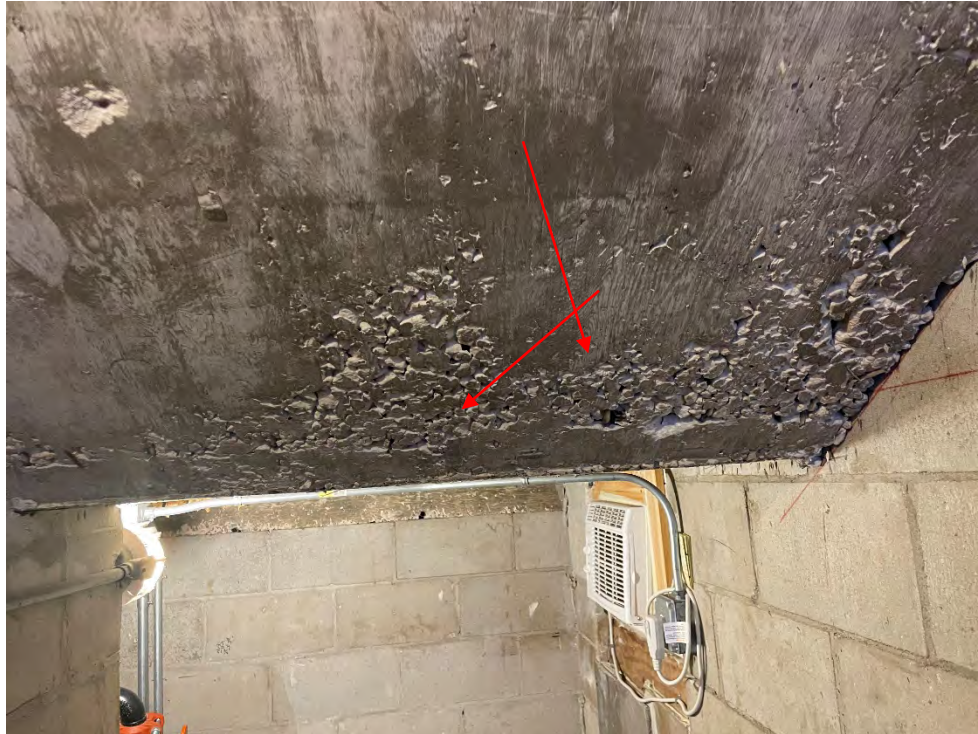
Figure 25 – Honeycombing of concrete in mechanical room
