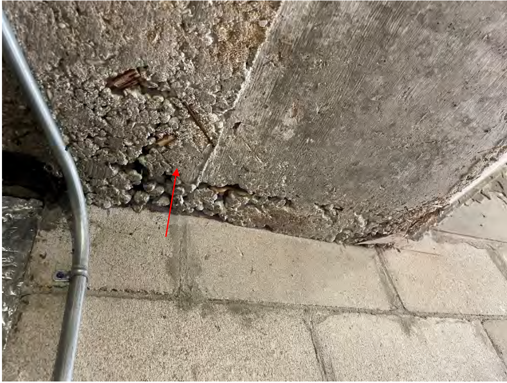
Figure 29 – Honeycombing in concrete in mechanical room
