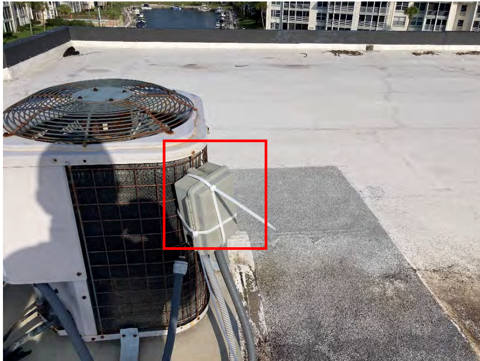
Figure 11 – A/C control box not properly secured
