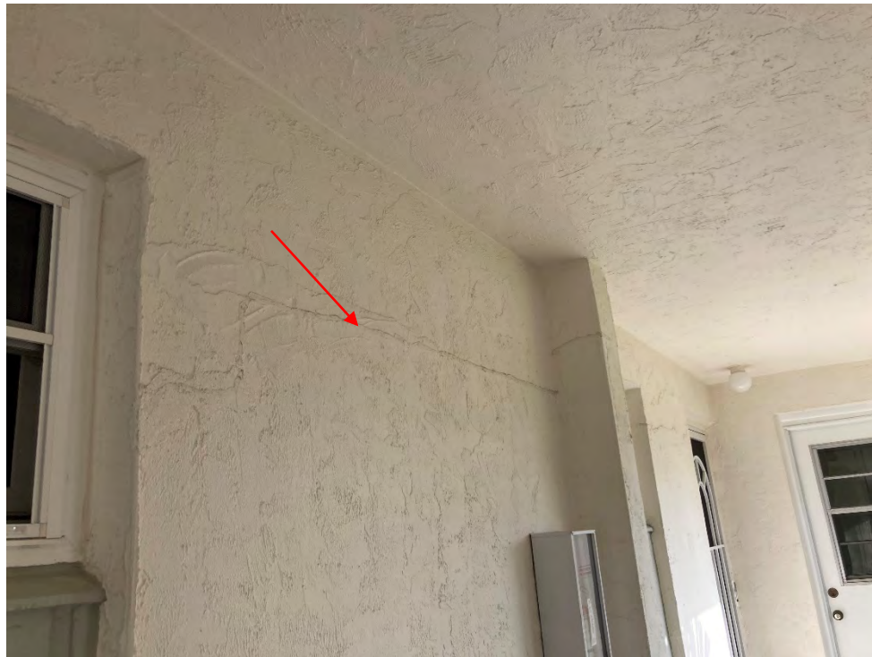
Figure 13 – Stairstepping on ground floor
