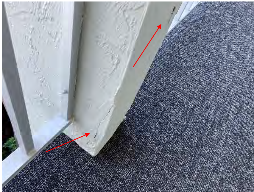
Figure 20 - Locations of potential spalling on column on 3 rd floor
