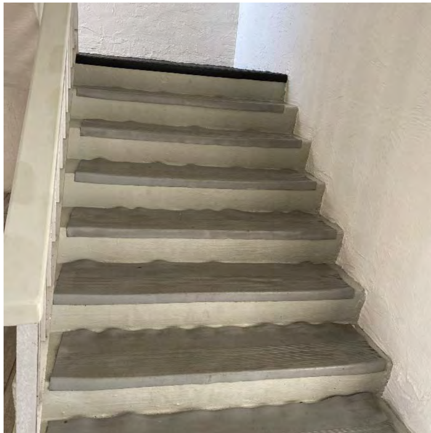
Figure 6 – Traction tracks on stairs starting to detach from stairs
