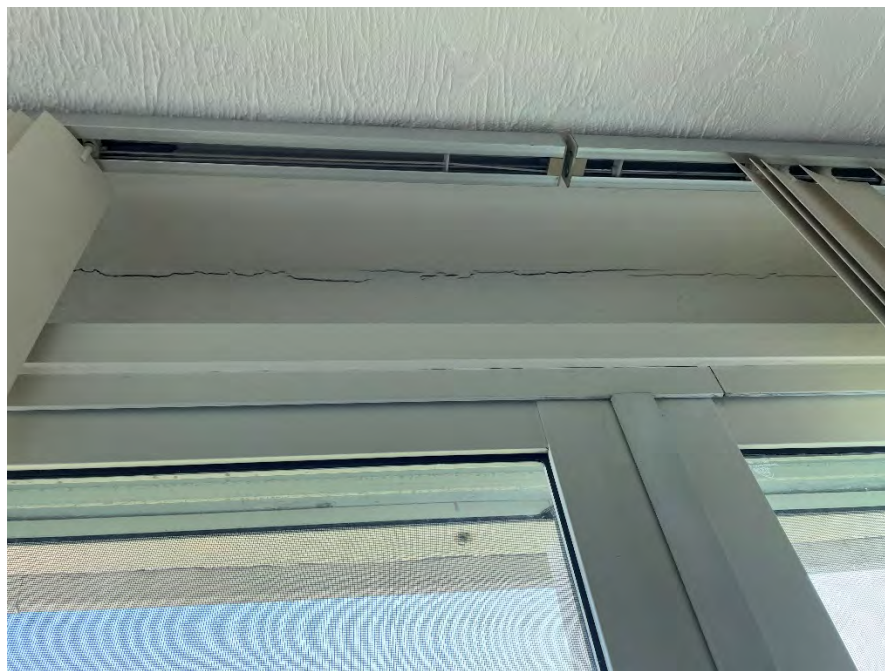
Figure 14 - Cracking of stucco and sealant in Unit E301
