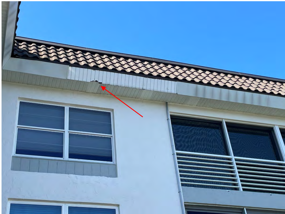
Figure 33 - Damaged fascia on exterior of the building
