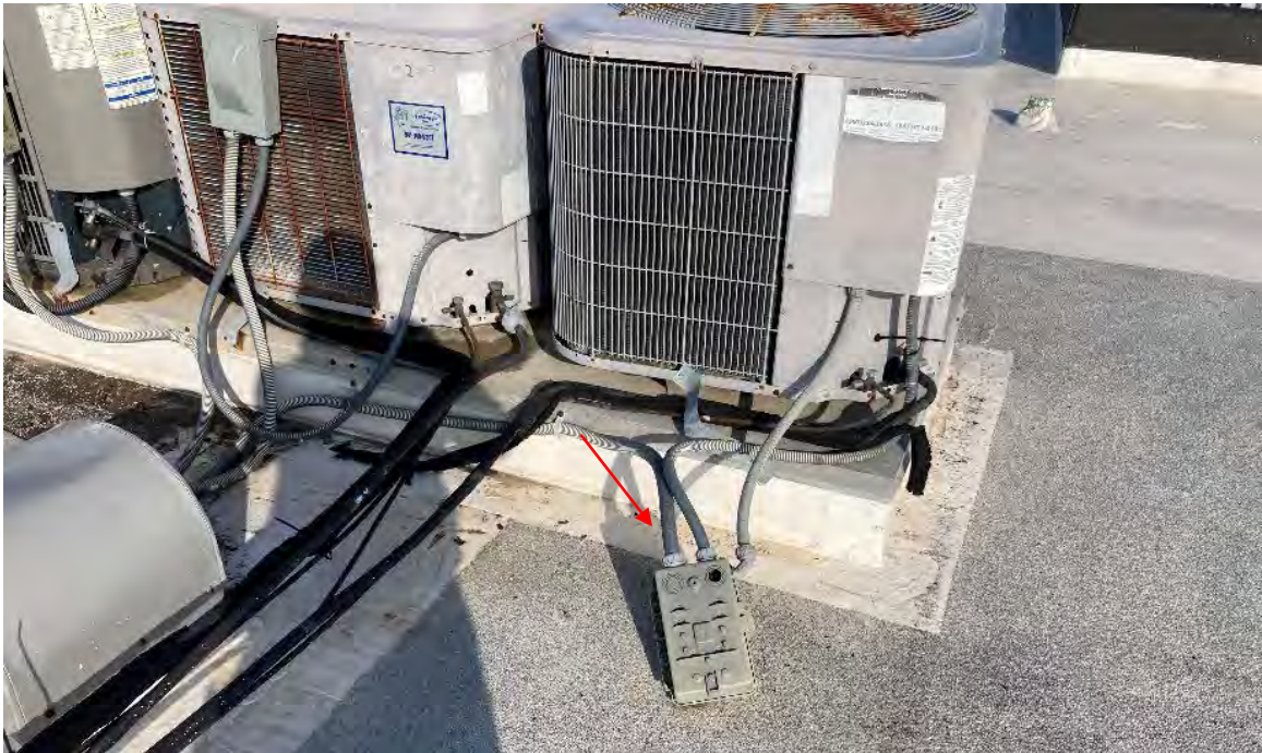
Figure 9 – A/C control box detached from unit
