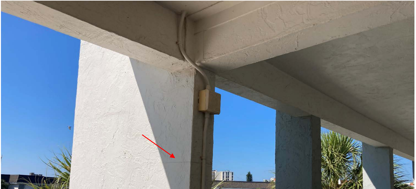
Figure 35 - Cracking on column on 3 rd floor
