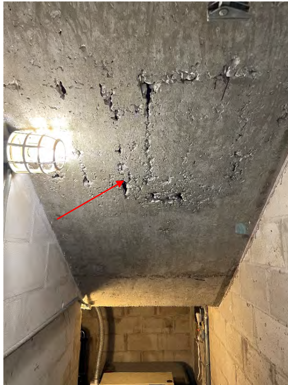
Figure 19 – Honeycombing of concrete in mechanical room
