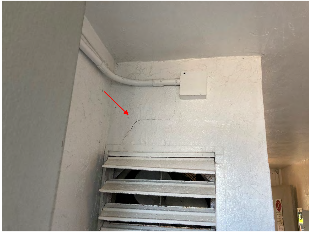
Figure 39 - Stair-stepping on ground floor
