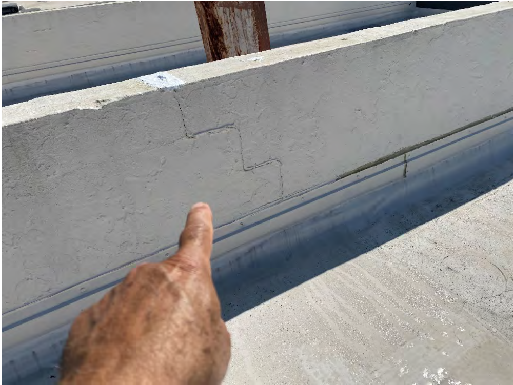
Figure 45 - Stair-stepping on parapet wall
