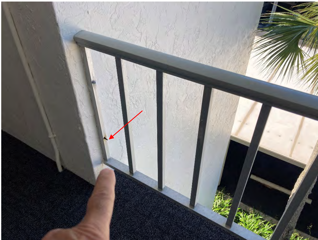
Figure 44 - Rusted walkway railing bolt on 3 rd floor
