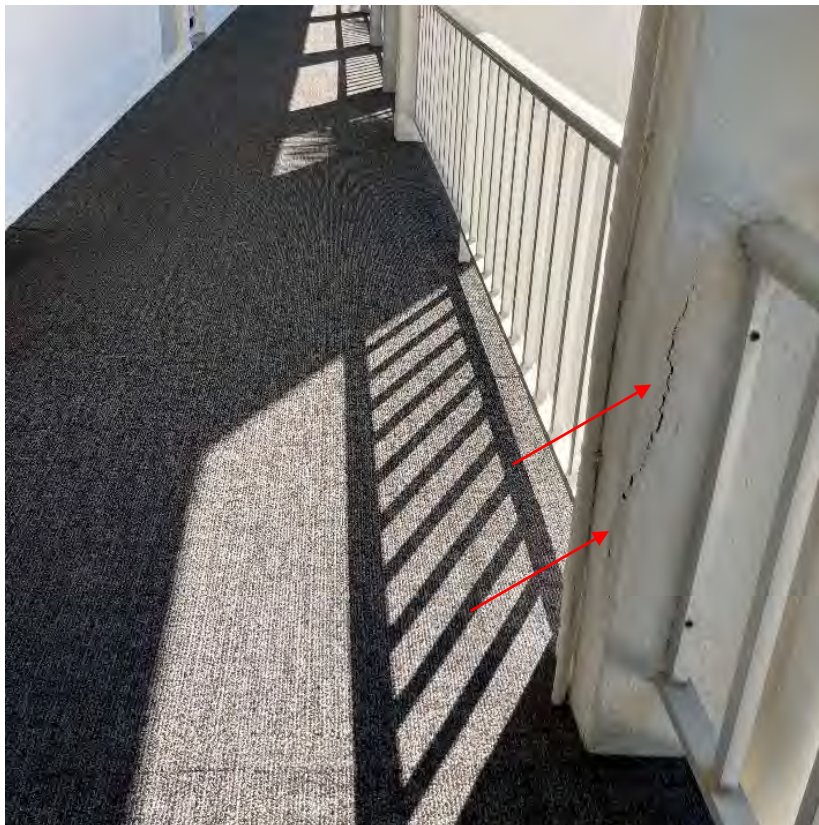
Figure 34 - Spalling on column on 3 rd floor
