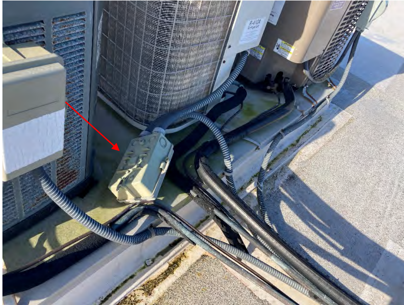
Figure 23 - A/C control box detached from unit
