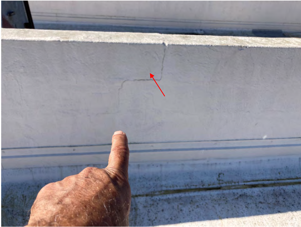
Figure 31 - Stair-stepping in rooftop parapet wall
