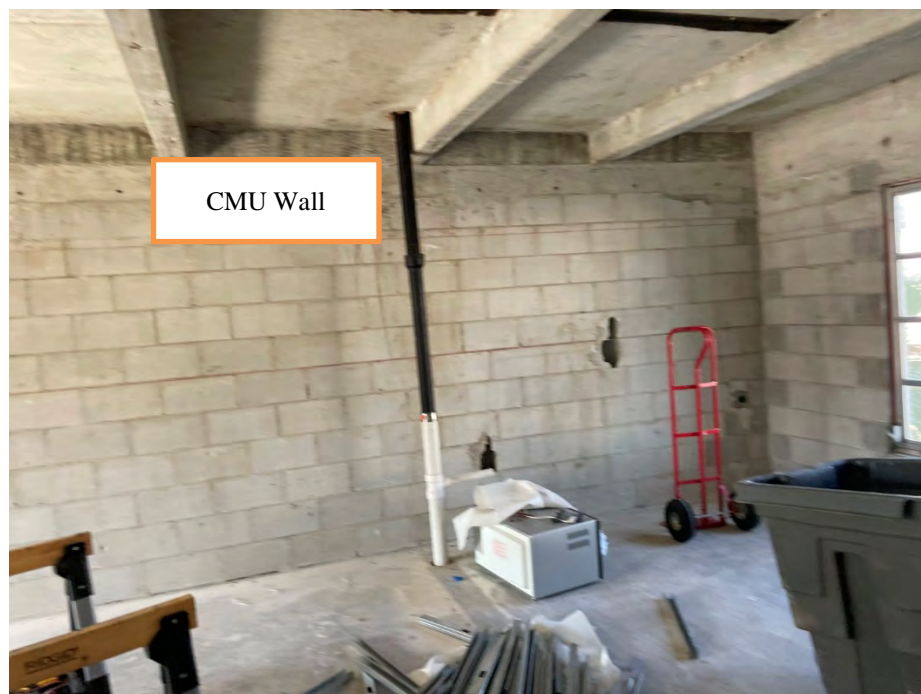
Figure 6: Example of CMU demising wall at Unit I 208
