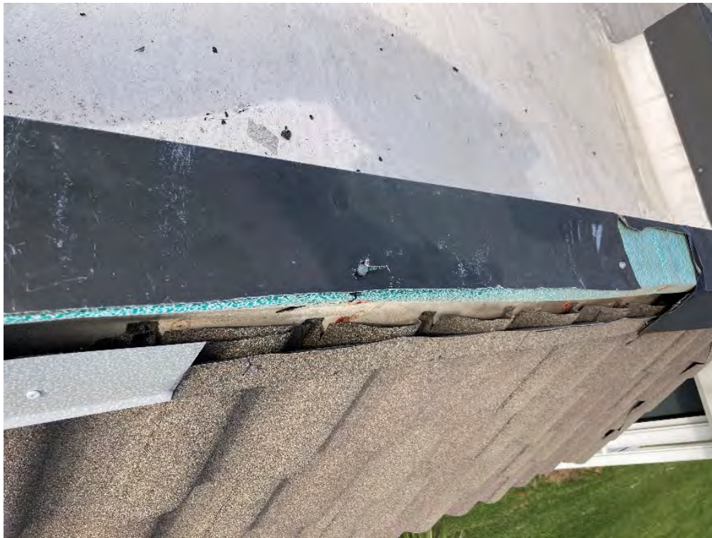
Figure 3 – Damaged coping along rooftop
