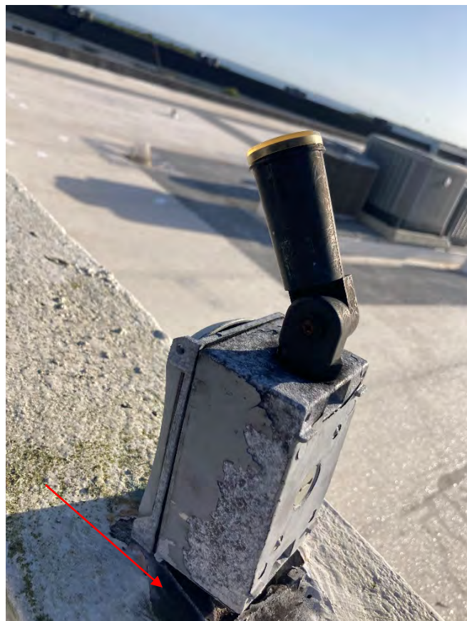
Figure 24 - Extrusion not sealed properly
