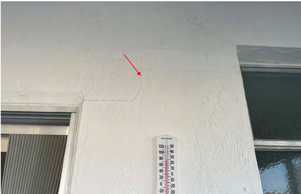
Figure 10 – Stair-stepping in Unit C202
