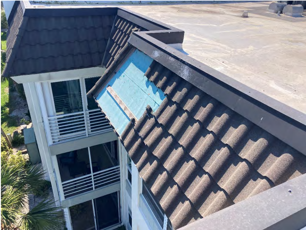
Figure 41 - Section of missing roof tiles
