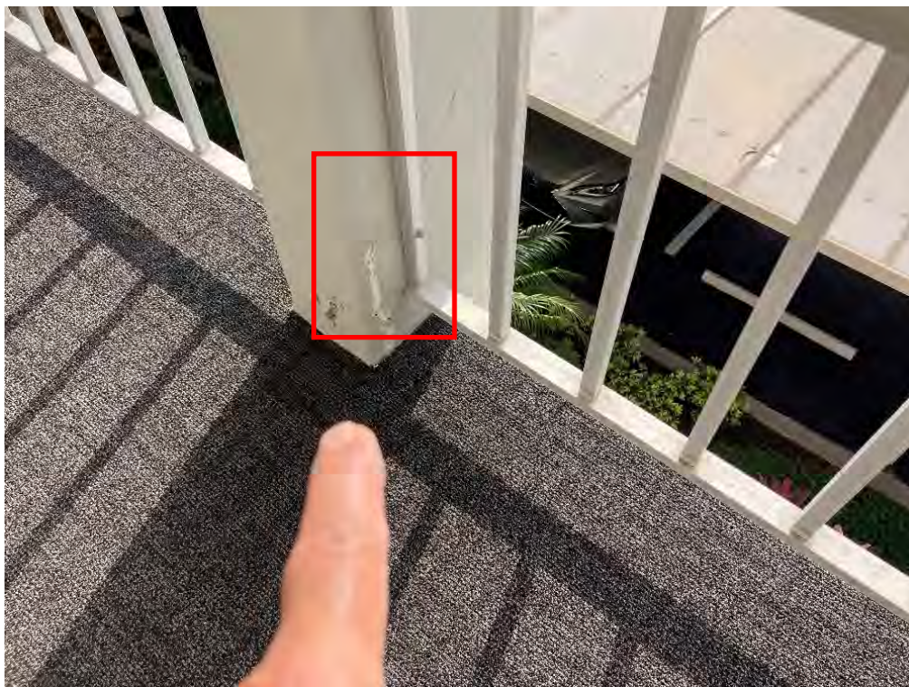
Figure 12 – Paint peeling on column
