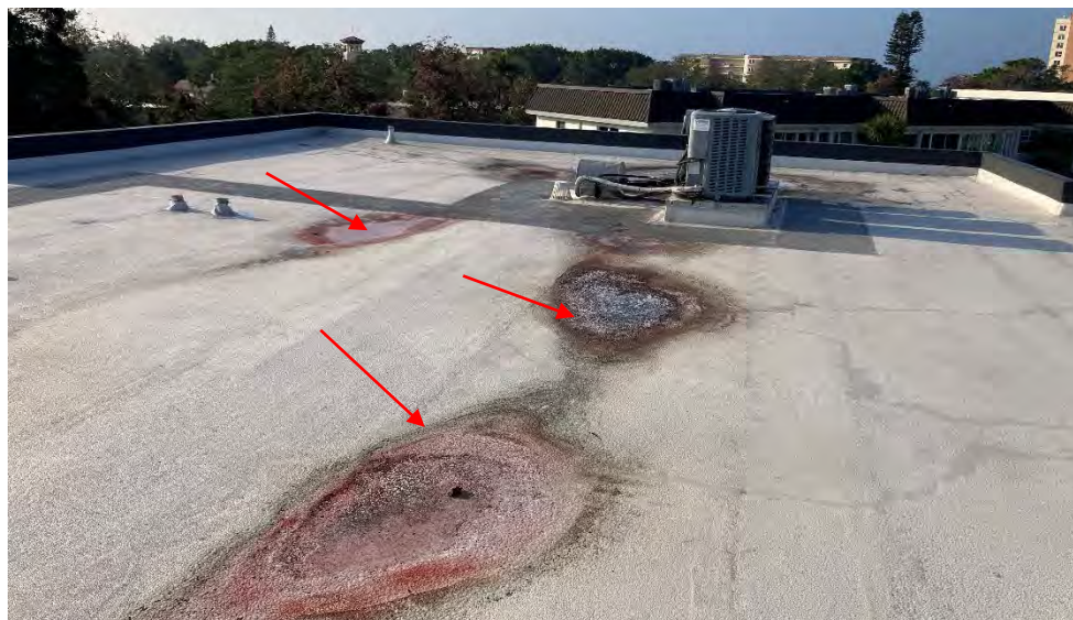
Figure 2 – Ponding residue on rooftops
