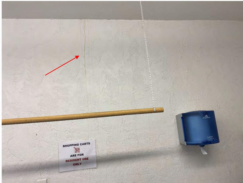
Figure 47 - Cracking on wall in laundry room
