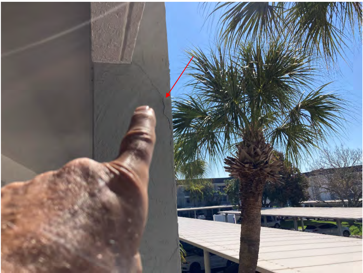
Figure 36 - Cracking on column on level two
