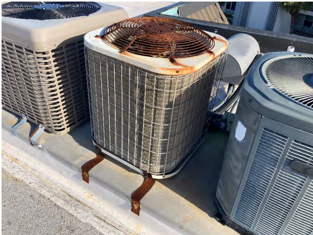
Figure 4 – Rusted A/C components
